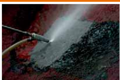
Surface - Sand Blasting
